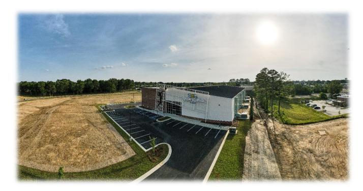
Beyond Construction completed this new 39,000 sf facility for Infinity Volleyball Academy in Brandon, MS. The project combined the use of multiple veneers, a partial parapet, a partial mezzanine, and integral structural steel framing to support a massive sign structure at the front of the building.
