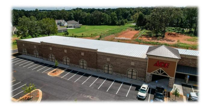
Stroud and Company recently completed this 22,145 square-foot commercial retail space for Ace Hardware and additional tenant space in McDonough, GA. The structure was created using two single slope metal buildings—79' X 196' and 59' X 103'.
