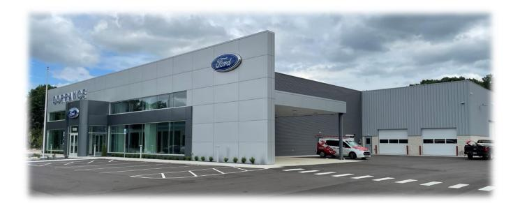
The facility features Kirby's Standing Seam 360 Roof System in galvalume. Kirby provided the extra column support for a storage space mezzanine. In addition to siding by others, the exterior utilizes Kirby's Reversed Roll Panel in pearl gray.
