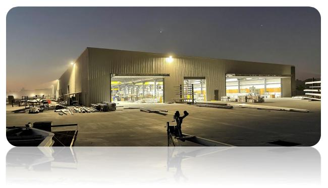
The boat trailer manufacturing facility is aesthetically pleasing with an exterior in the Kirby Standing Seam 360 roof system in Galvalume and the KirbyRib II wall panel in Fox Gray.
