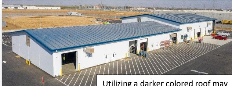
Utilizing a darker colored roof may not meet the roof solar reflectance and thermal emittance values specified in IECC and ASHRAE 90.1 codes.
