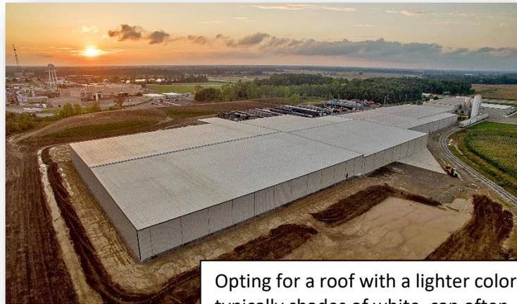
Opting for a roof with a lighter color, typically shades of white, can often meet the reflectance and emittance values required.
