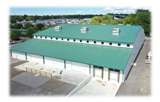
The facility features a 150'  $\times$  150' main building and a lean-to on each side, both 40'  $\times$  150'. The building utilizes the Kirby SS360 Standing Seam roof system and KirbyWall panels.
