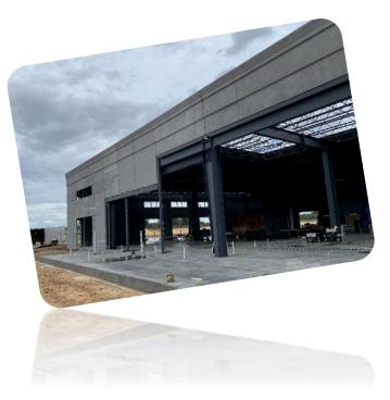
horizontal tube along the wall of areas with an adjacent lower roof. These large rectangular tubes support pre-cast walls above the adjacent roof areas.
