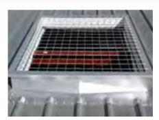
6. Welded safety frame is ready for Prismatic Skylight.
